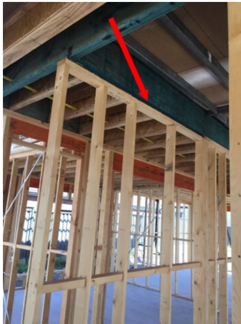
FIGURE 2.2 FIXING OF TRUSSES TO FREESTANDING NON-LOADBEARING WALL THAT IS A BRACING WALL
